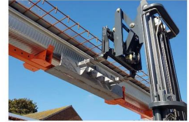
2019 - ongoing Platform 3 - Landsec 'The Forge'
